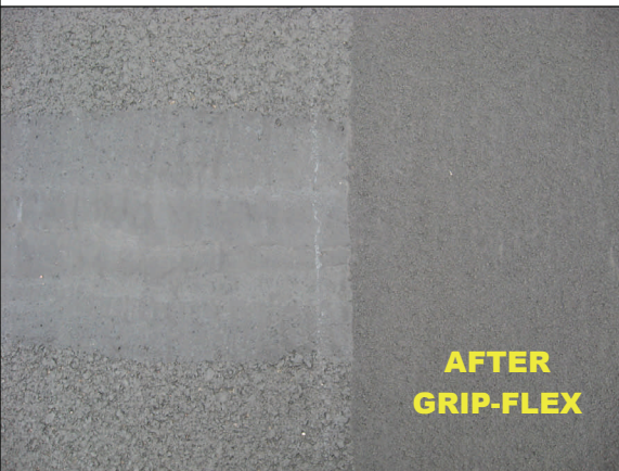
Below: Crack Filled with GRIP-FLEX Crack Fill and partially covered with GRIP-FLEX Surfacing
