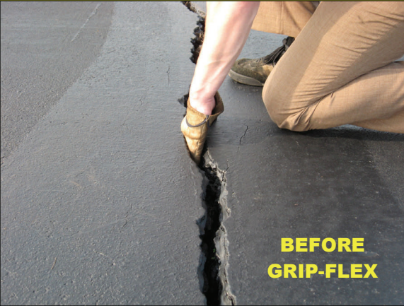
Above: Very Deep Wide Crack at Tulsa Riverside Airport:
